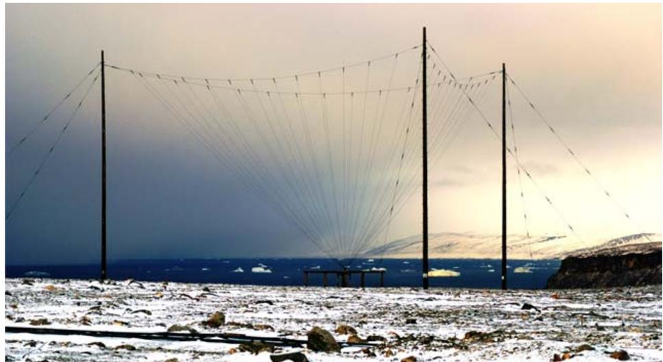
The inverted discones can be used as low as 80m and 160m, using a tuner.
