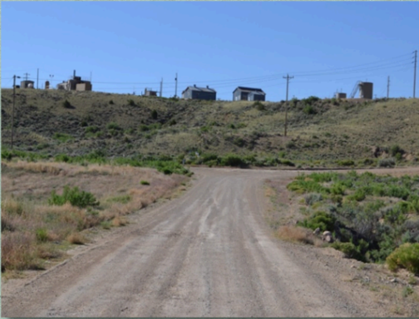
Turn right at pumping station.
